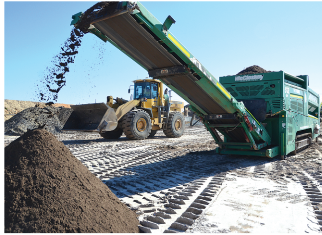
Biopiles under construction at Eclipse Soils resource recovery centre
